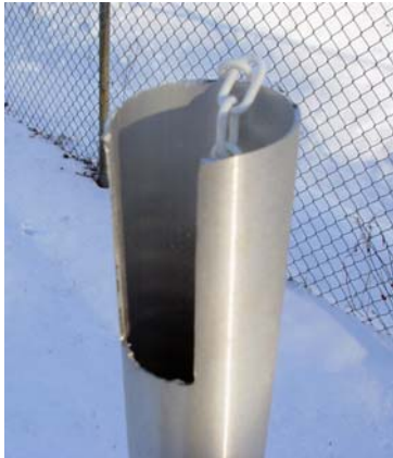
Broken sections of an aluminum flagpole
